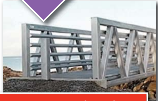
The Quaqtq bridge in northern Quebec, Canada is a pony-truss bridge made of 6061-T6 aluminum extrusions. Courtesy of MAADI Group Inc.
