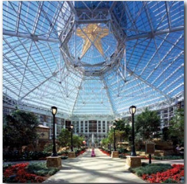
Photo courtesy of Naturalite Skylight Systems by The Vistawall Group. Photographer: Wes Thompson.
